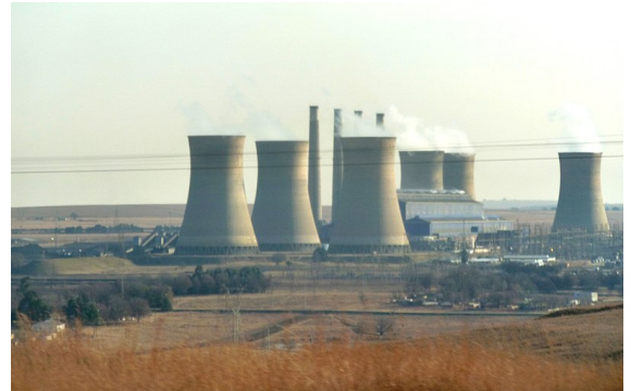
Camden Power Station, South Africa. Photo: JMK (Creative Commons, 2017)
