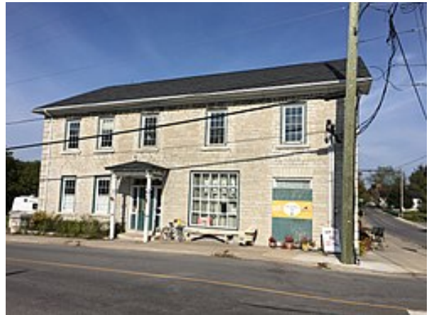
The limestone building that housed a series of general stores (photo: kermitchemist, Creative Commons, 2019)
